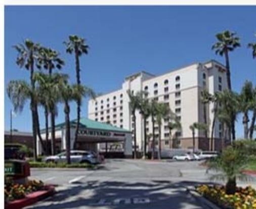
Courtyard by Marriott Baldwin Park
